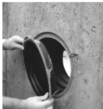
6. After the concrete is poured and cured, remove end caps with screw driver or crow bar. End caps may be replaced to protect sleeve until pipe penetration is made.
